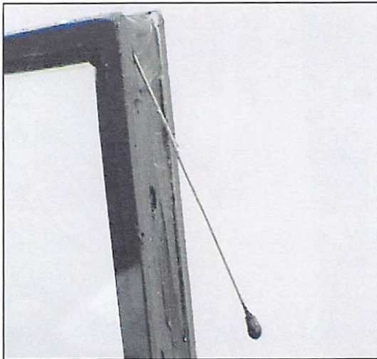
2. Apply a dab of silicone sealant at the end of the capillary tube after it has been cut.
