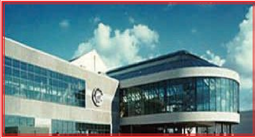
Carousel Center, Syracuse, NY, Dal Pos Architects, PPG Solex and Sungate 100 Low-E Insulating Glass
